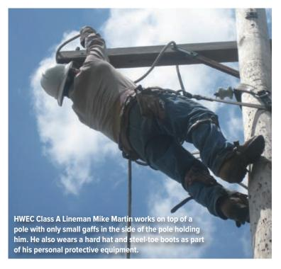
"hardheaded" our linemen are, they still need protection. Insulated hard hats are worn at all times to protect them from blows and falling objects.
